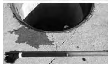
Inspection Utilizing Sediment Probe
