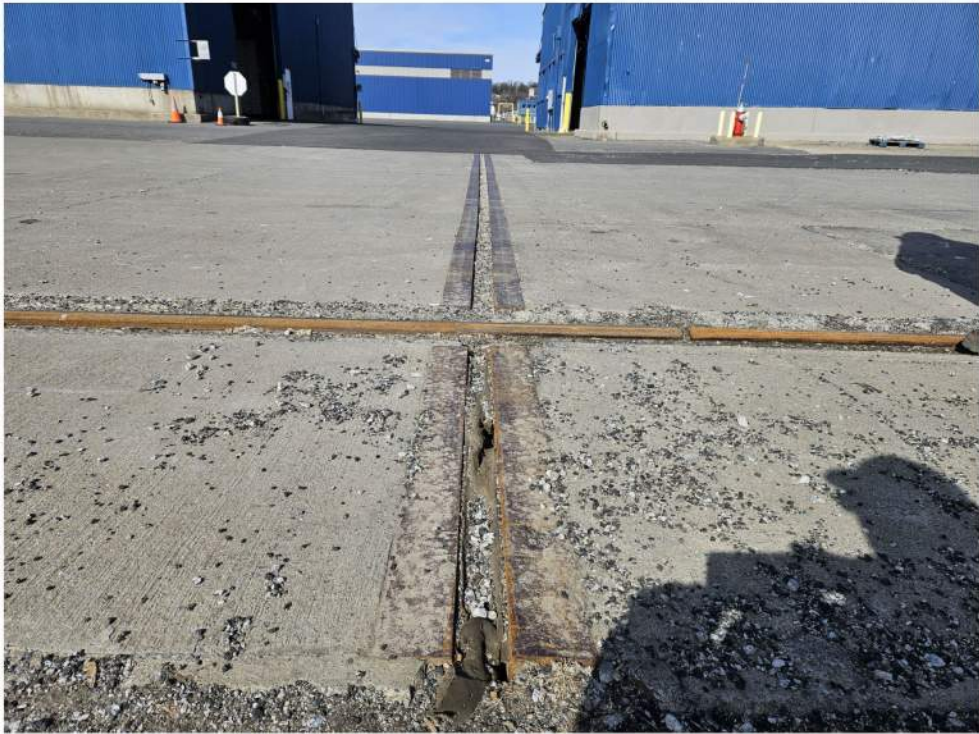
Tags:Topside, Report Photos Taken by:Anthony DeVito Date taken:03/12/2025 Media 4: Bent 1 Expansion Joint
