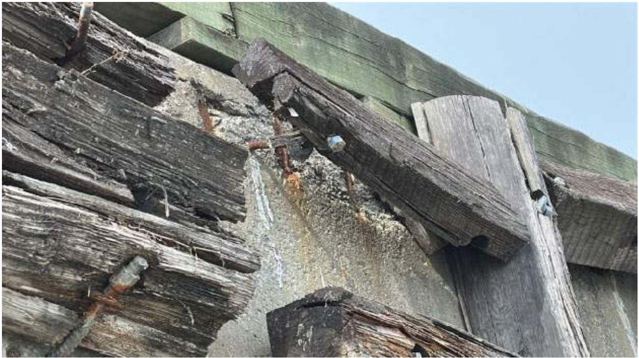
Tags:Fendering, Report Photos Taken by:Matthew Seinuk Date taken:03/12/2025 Media 237: Exposed rebar on fascia beam between bent 52 and 53
