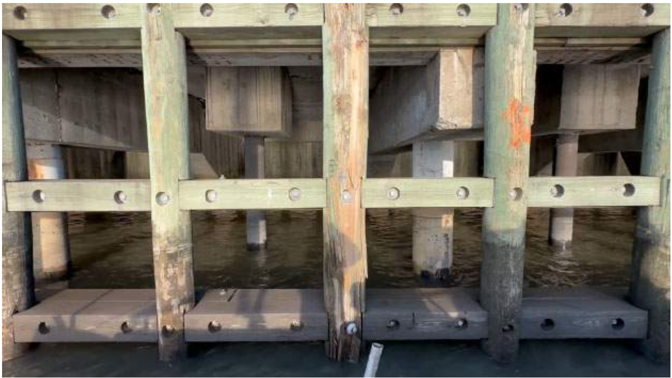
Tags:Fendering, Pile Caps Taken by:Anthony DeVito Date taken:03/24/2025 Media 21: Bent 9, P-9
