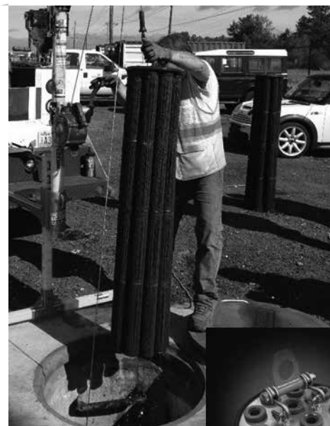
Cartridge Removal & Lifting Device
