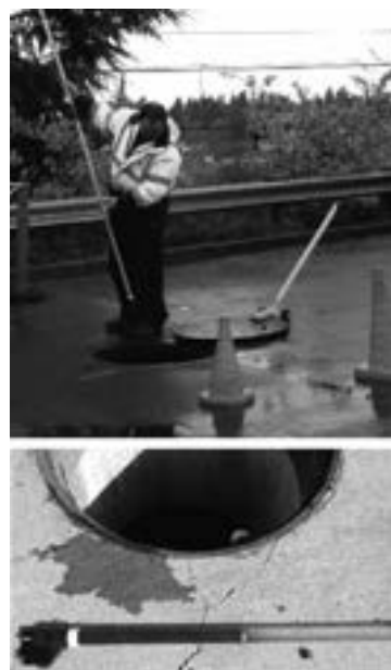
Inspection Utilizing Sediment Probe
