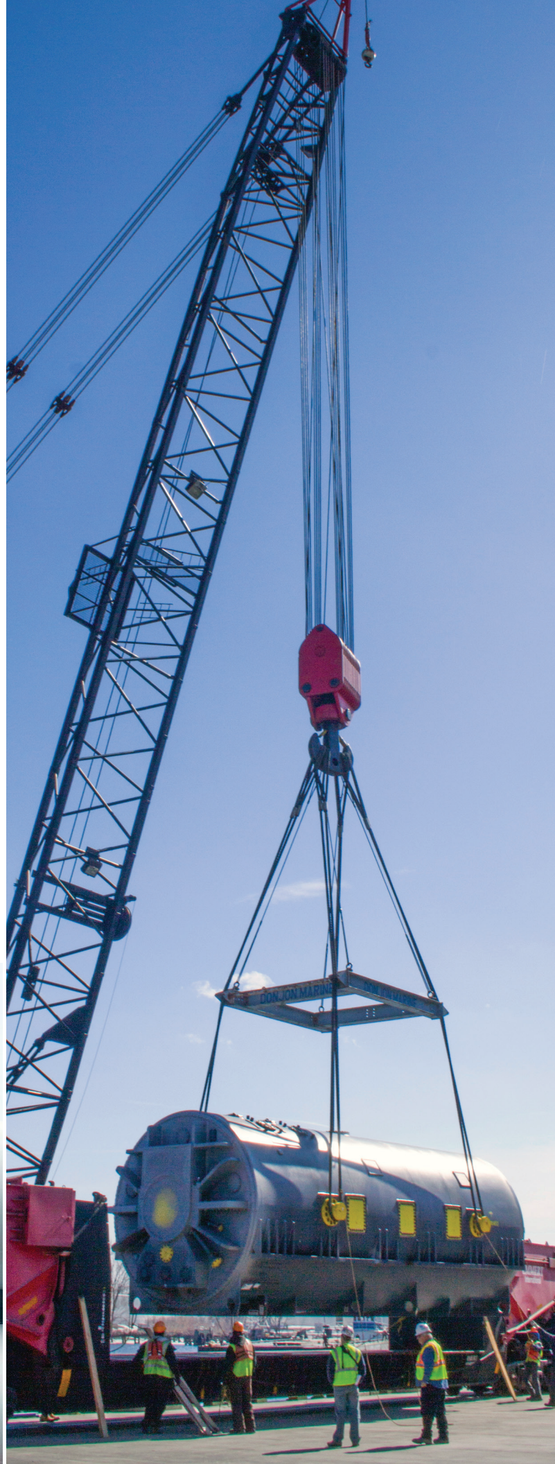
FMT longshoreman unloading wind blade shipment from the BBC Arizona that arrived at the Port of Albany from Brazil. The blades are destined for a wind energy project in western NY.
