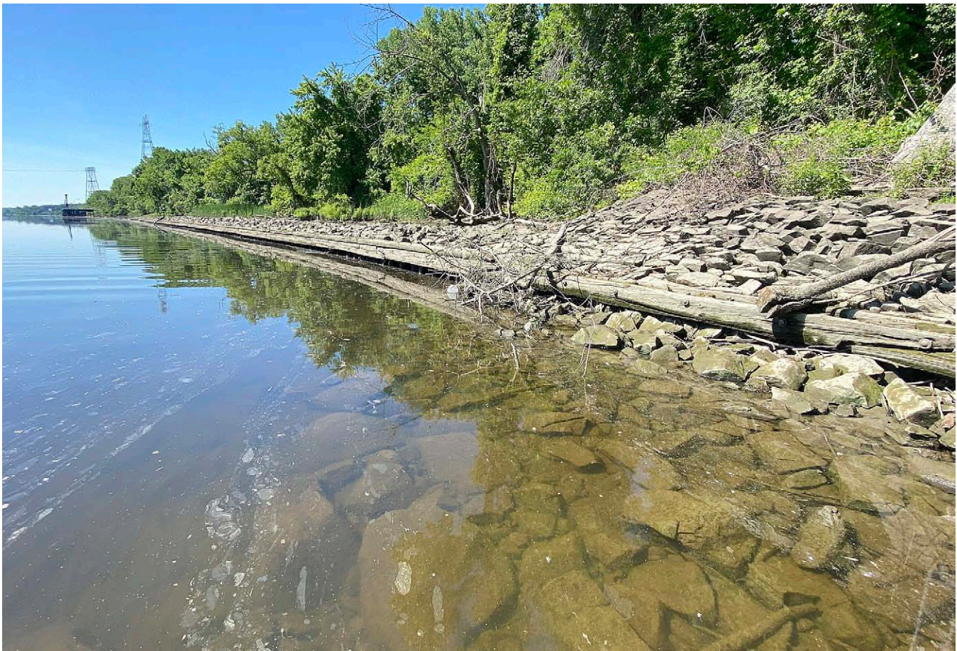
Hudson River shoreline along the proposed Port of Albany development project.
